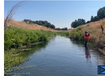
A5 – Bank-protected canal. Gentle slope, artificial bank composition, and fine bed sediment
