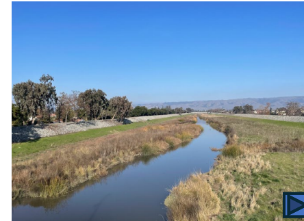
A6 – Ditch. Low to moderate entrenchment, gently sloped, natural bank composition, plane bed, fine bed sediment
