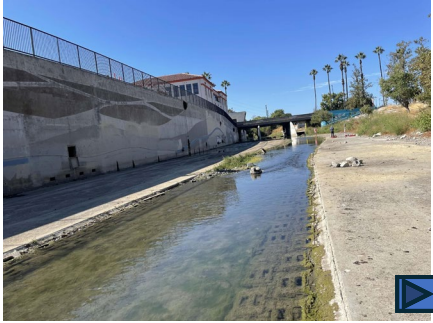
A2 – Bank-protected river. Steep, artificial bank composition, mixed-size natural bed composition including coarse sediment
