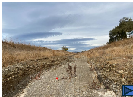
A3 – Naturalizing canal. Deeply entrenched, wide, natural bank composition, strong bed undulations, coarse bed sediment
