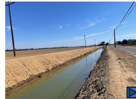
A6 – Ditch. Low to moderate entrenchment, gently sloped, natural bank composition, plane bed, fine bed sediment
