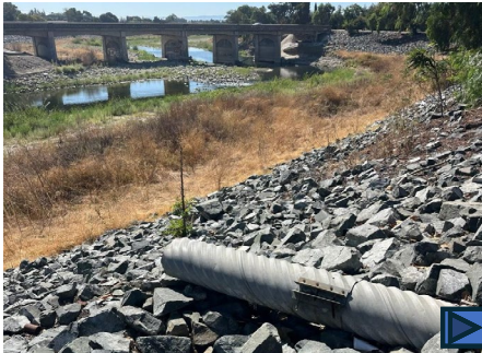
A3 – Naturalizing canal. Deeply entrenched, wide, natural bank composition, strong bed undulations, coarse bed sediment
