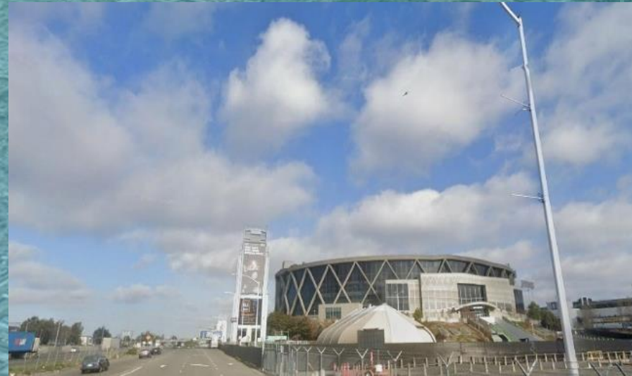
Bridge at Coliseum
