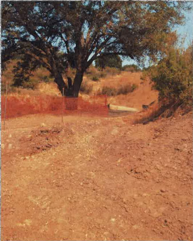
CLEARING, GRUBBING, ROUGH GRADING: STREAM CHANNEL 22; FACING WEST
