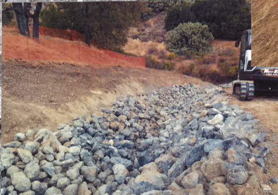
RIP RAP INSTALLATION: STREAM CHANNEL 31: FACING NORTH
