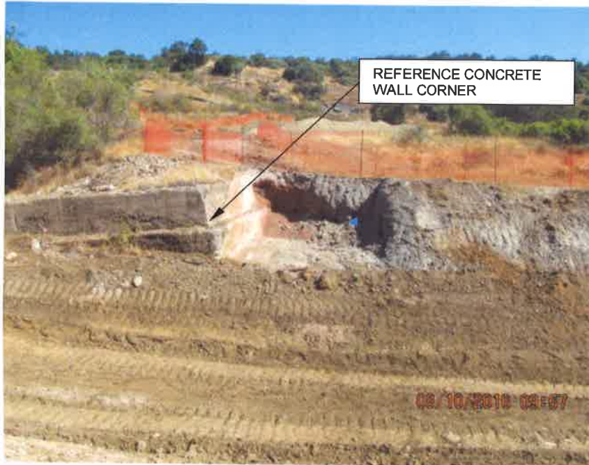
McAbee Creek – Looking north from south bank of creek at the additional calcine excavation adjacent to the concrete wall. This excavation is at Senador Mine Trail.
