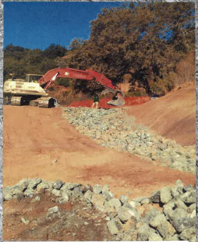
RIP RAP INSTALLATION: STREAM CHANNEL 22; FACING WEST
