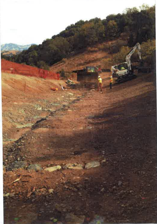
SENADOR MINE RESTORATION PROJECT, SANTA CLARA COUNTY PARKS
