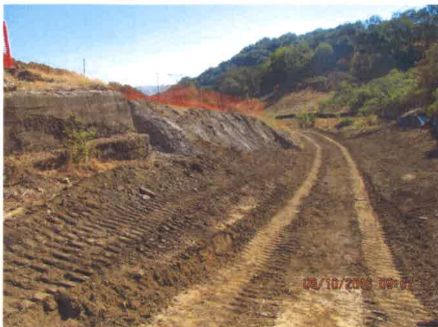
McAbee Creek – Looking downstream from above TF 45. Gray area on the left (north bank) has been excavated to remove calcines. The concrete wall is shown on the left side of the photo.
