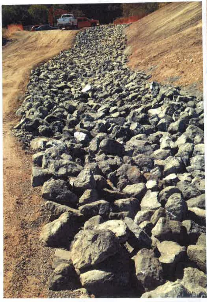
RIP RAP INSTALLATION: STREAM CHANNEL 22; FACING WEST
