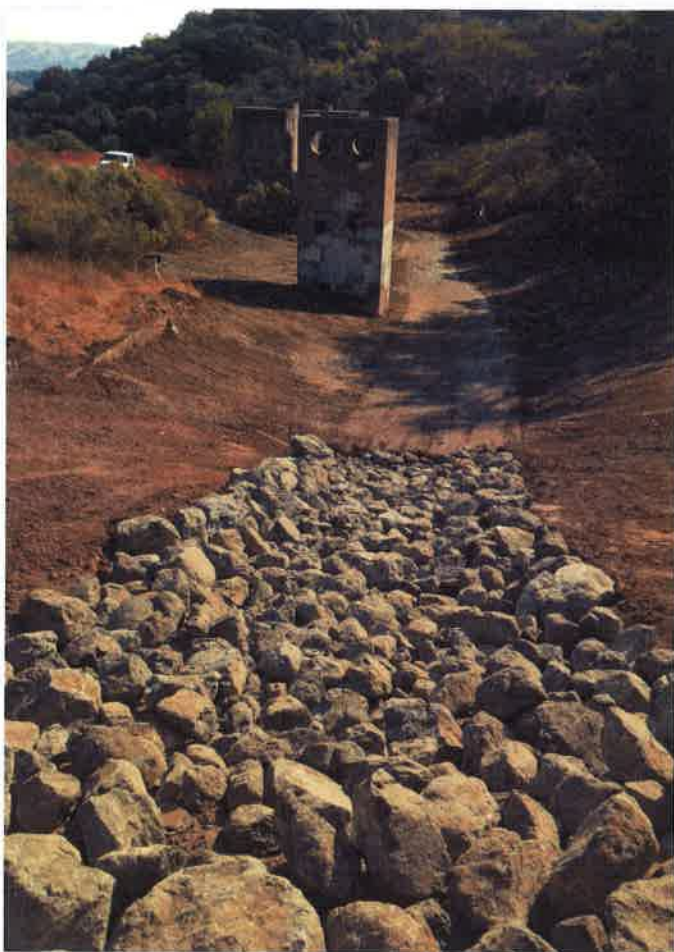
RIP RAP INSTALLATION: STREAM CHANNEL CC/CD/45; FACING EAST
