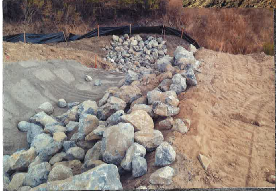
RIP RAP INSTALLATION: STREAM CHANNEL 31: FACING NORTH
