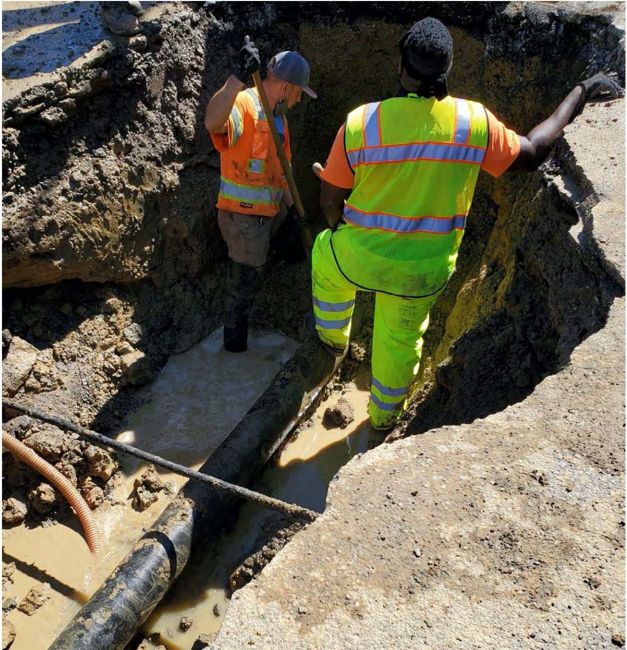
A broken pipe main in Marin City from Fall 2020 at the intersection of Phillips Drive and Drake Avenue. The break closed down a church and a school for a week as water overflowed. Photo: Terrie Green
