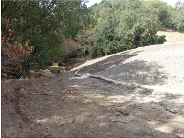
Photo point 4 sequence. Slope flattening through erosion control completion.
