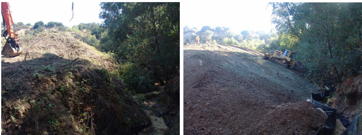
Slope flattening to achieve stable slope configuration.
