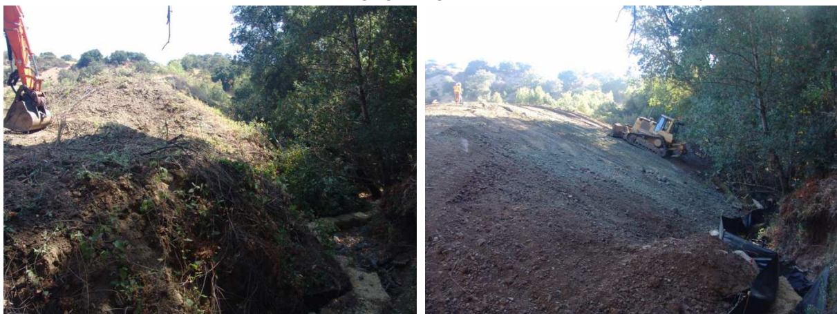
Figure 3. Slope flattening to achieve stable slope configuration.
