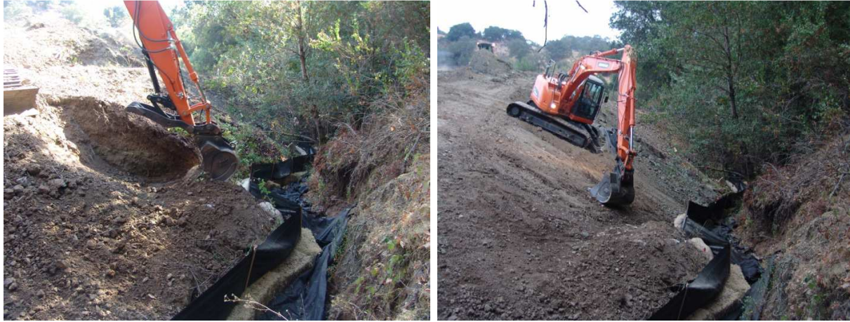
Creek protection BMP's.
