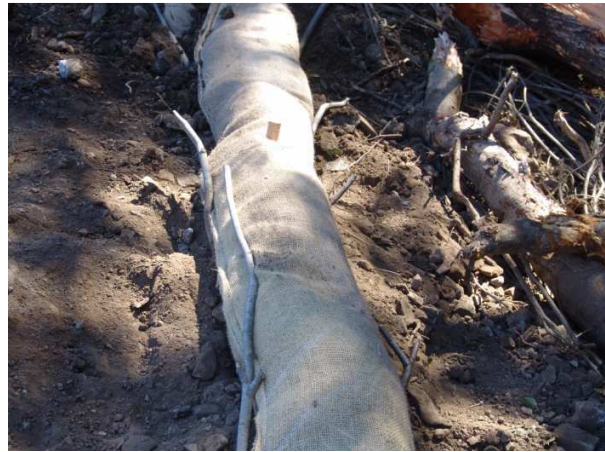
Willow poles planted in straw wattle trench.
