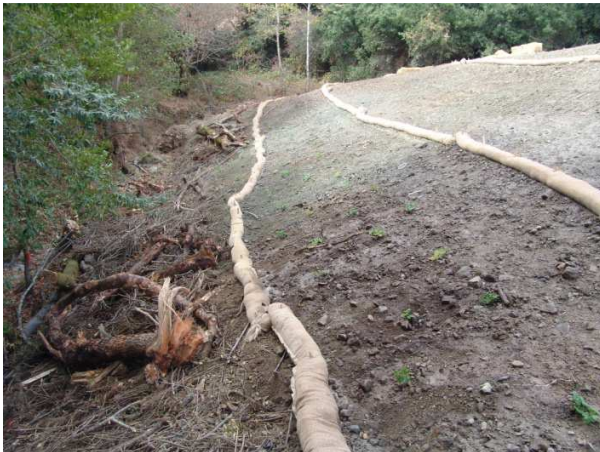
Photo point 5 sequence. Slope flattening, creek-side restoration, final erosion control implementation.
