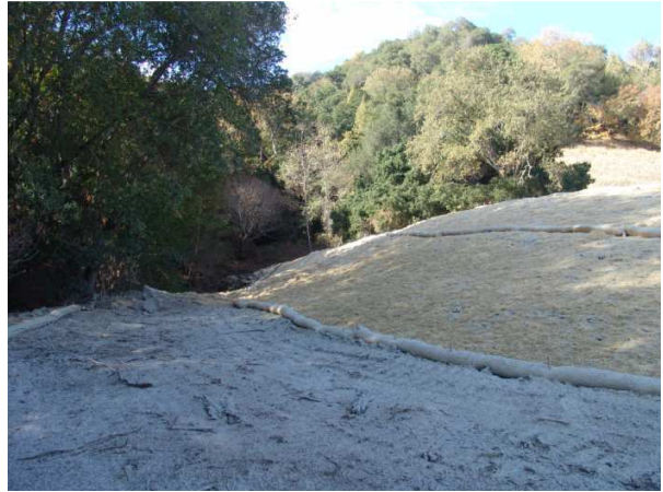
Figure 10. Photo point 4 sequence. Slope flattening through erosion control completion.
