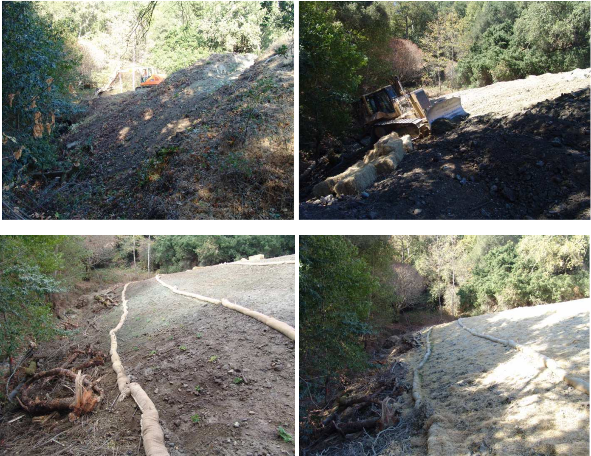
Figure 9. Photo point 5 sequence. Slope flattening, creek-side restoration, final erosion control implementation.
