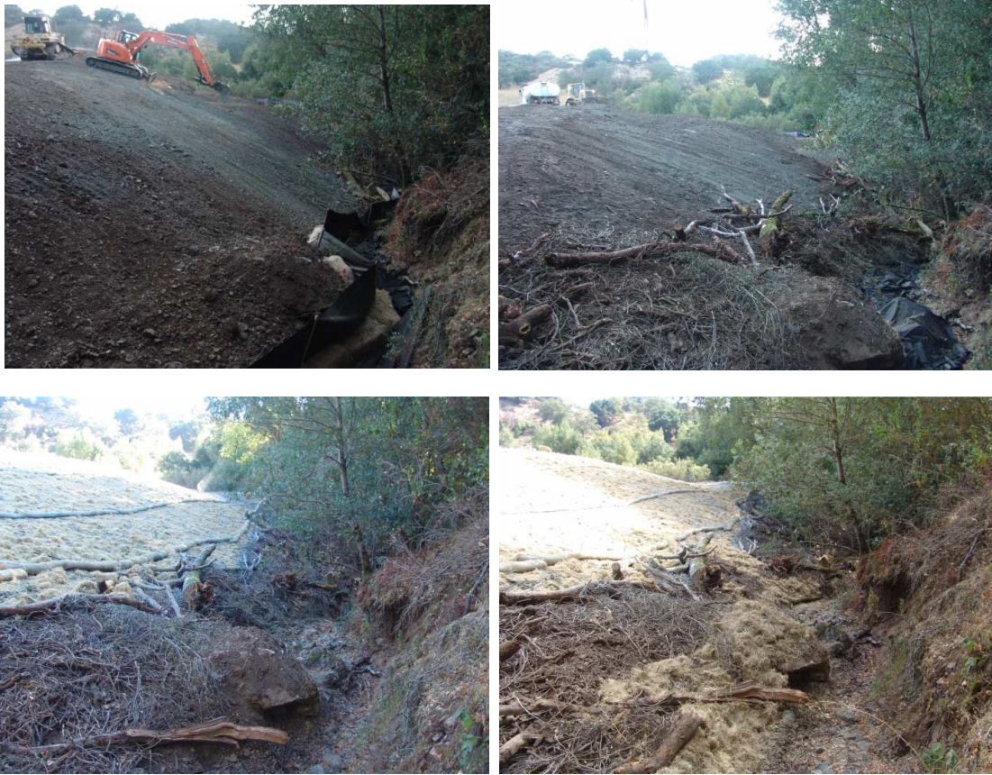
Figure 6. Creek protection, restoration.
