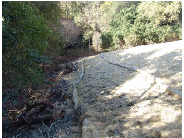
Photo point 5 sequence. Slope flattening, creek-side restoration, final erosion control implementation.
