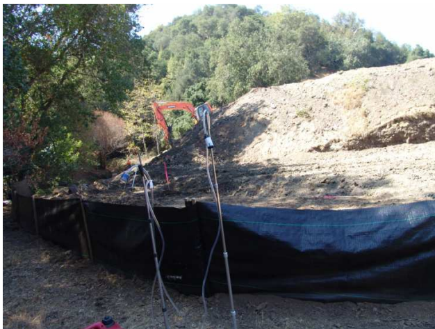
One of four perimeter air monitoring locations.
