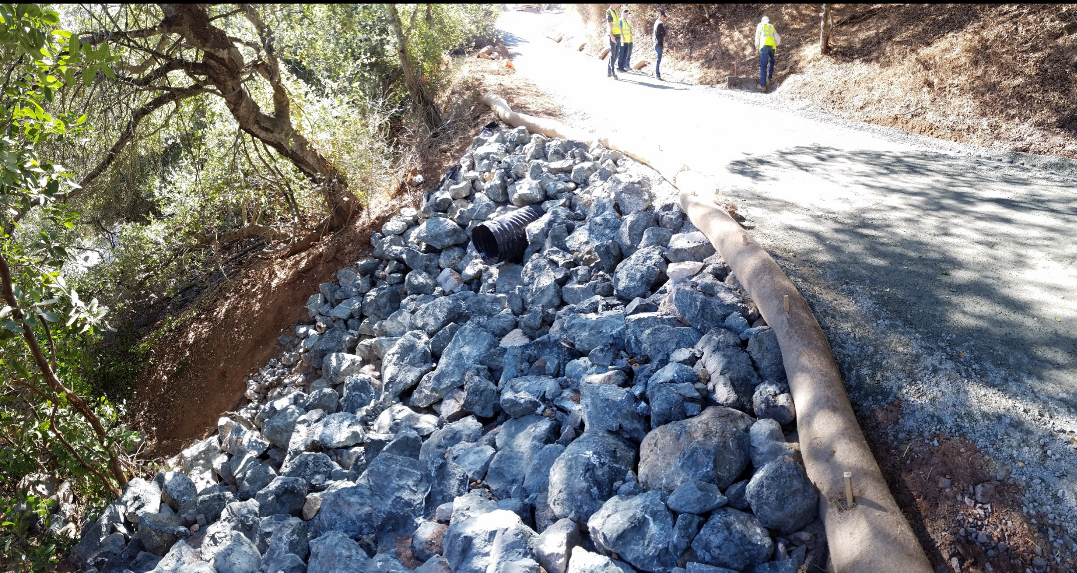
New corrugated culvert pipe installed on Yellow kid Trail with outfall erosion protection.
