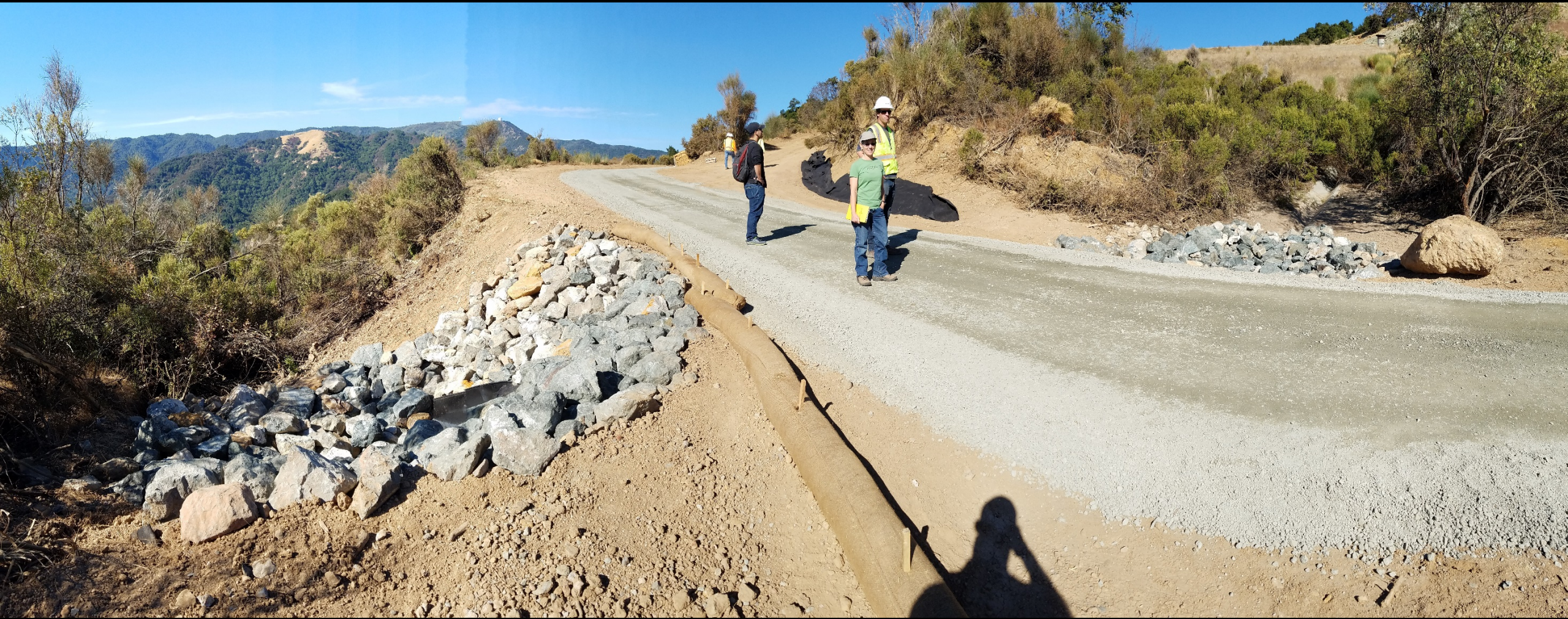
Waterboard and Roux consultants examine a culvert drainage upgrade on Castillero Trail. All calcines have been removed at the time of this photo.
