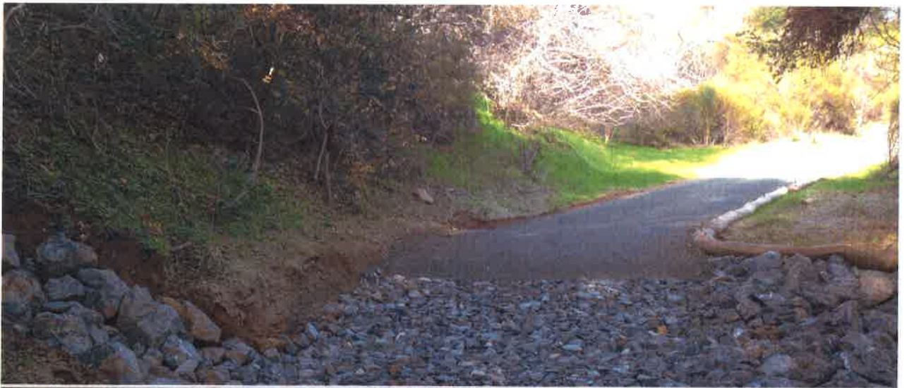
Yellow Kid Armored Crossing
