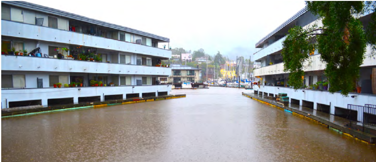
Flooding in the Canal area.
