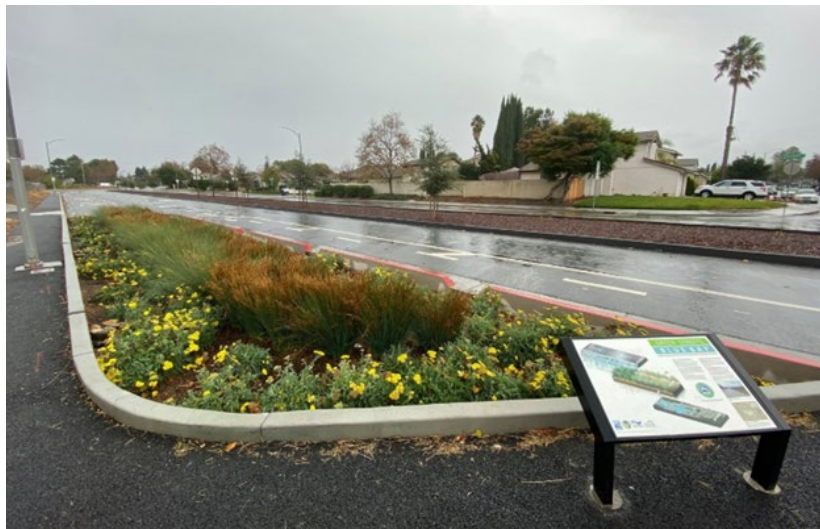
Green Stormwater Infrastructure Installed on Chynoweth Ave, San Jose
