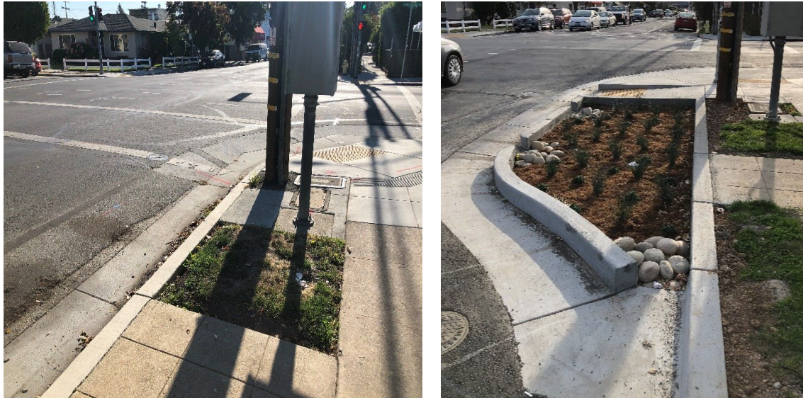
Before and After of GSI Retrofit in San Mateo Residential Neighborhood Intersection
