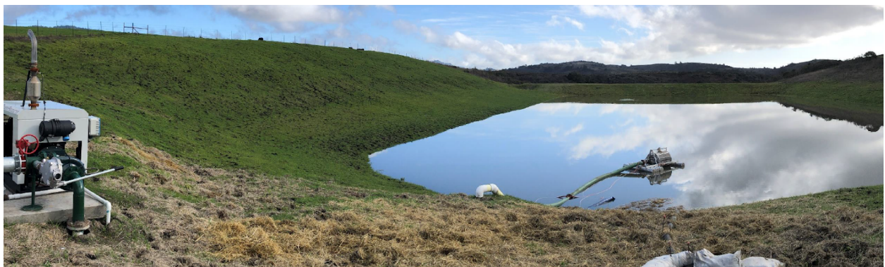
New water storage pond on Butano Farm. Photo Credit: Jarrad Fisher
