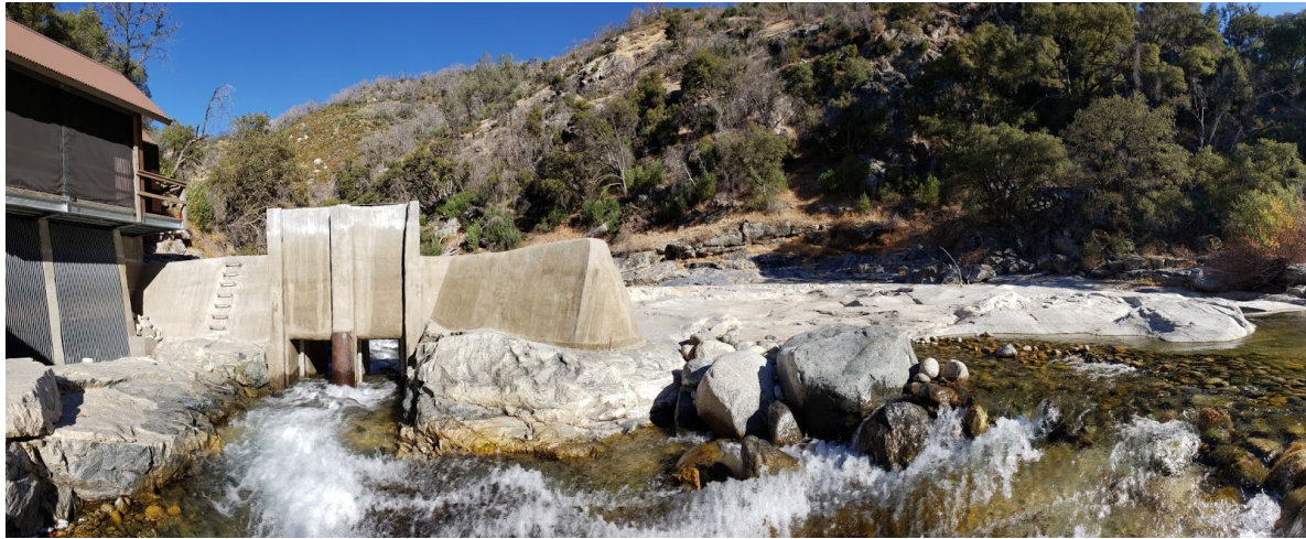
Lower Cherry Creek dam diversion structure. Photo Credit: James Muller
