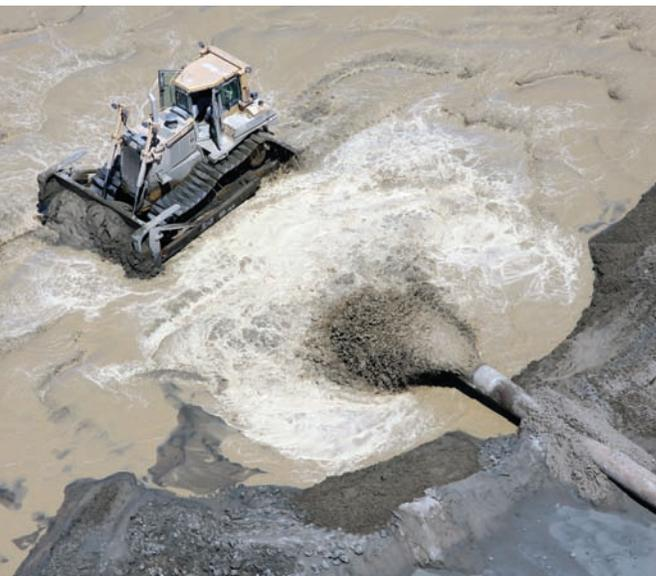
Dredged sediment from the Port of Oakland being used to build up Hamilton Wetlands. Photo courtesy of Manson/Dutra Joint Venture.
