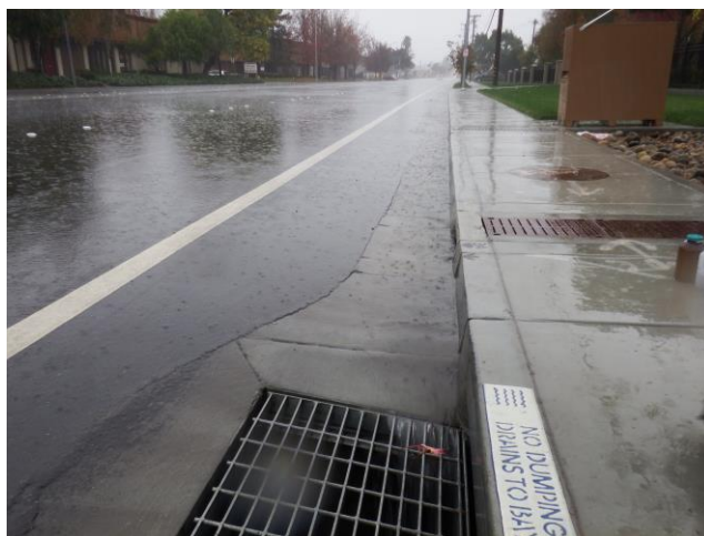
Figure 8. Stormwater bypassing the TWF inlets and flowing directly into the storm drain untreated was observed during storm events with rainfall intensities of 0.33 in/hr and greater.
