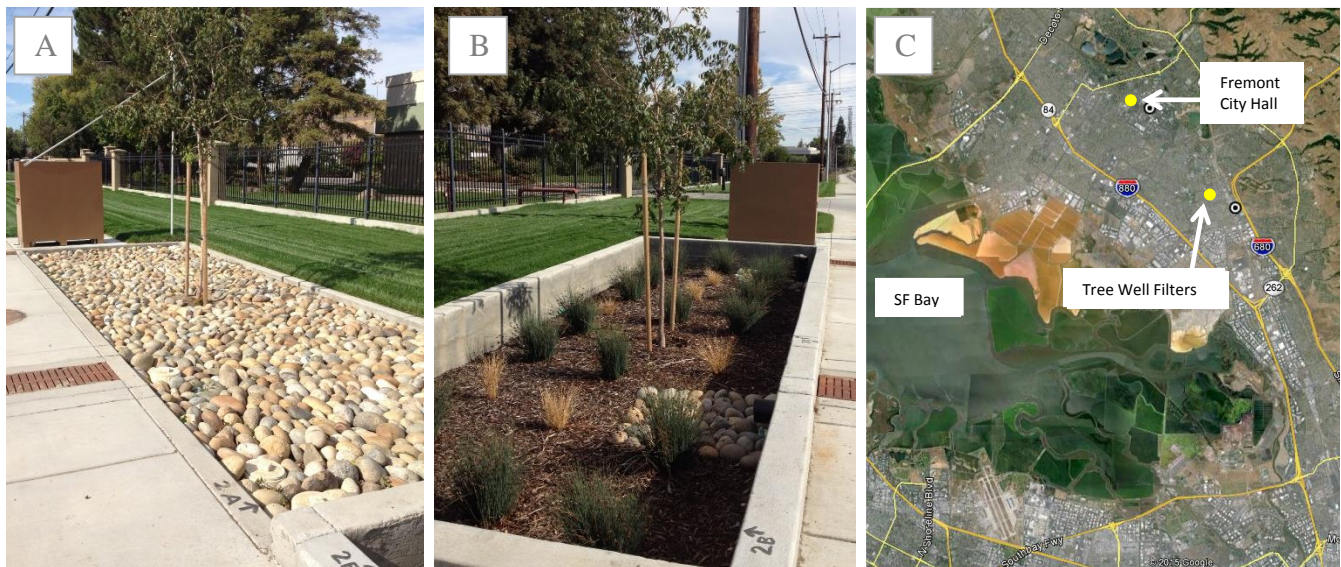
Figure 1. A) Subsurface-loaded tree well filter, B) surface-loaded tree well filter, and C) regional aerial of southeast and South San Francisco Bay showing location of tree well filters in the urban Fremont area.
