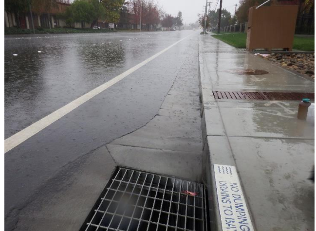
Figure 4. Stormwater bypassing the subsurface-loaded TWF inlets and flowing directly into the storm drain via the adjacent drop inlet
