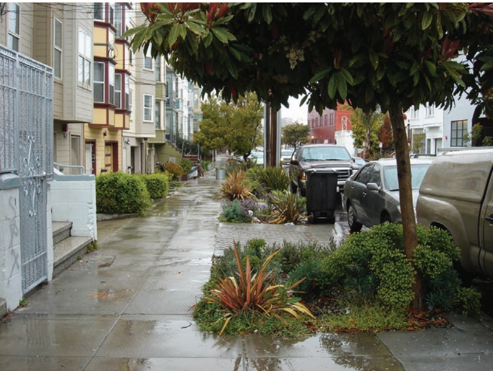
Shotwell Street, San Francisco: after. Plants filter and slow runoff. Photo courtesy of plantsf.org.
