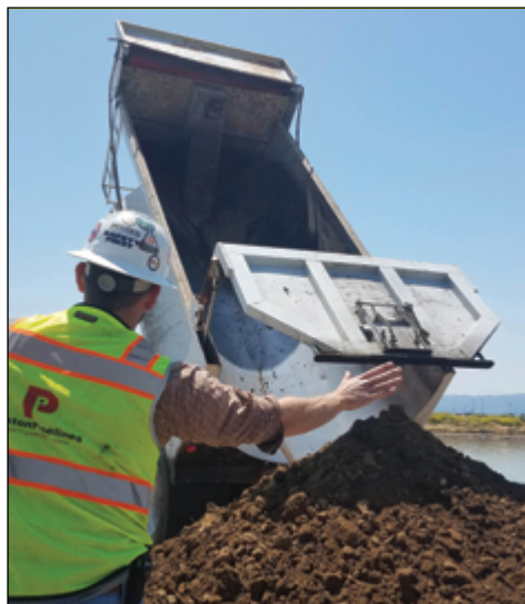
Stockpiling dirt in advance of shoreline project at Alviso site. May 2019. Photo courtesy USCOE
