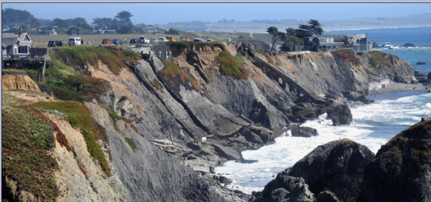
Erosion threatens cliff-top buildings in Sonoma County. Photo: Jacoba Charles
