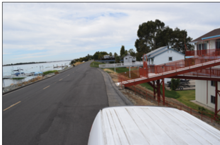
Subsided homes on Brannon Island. Photo: Amber Manfree
