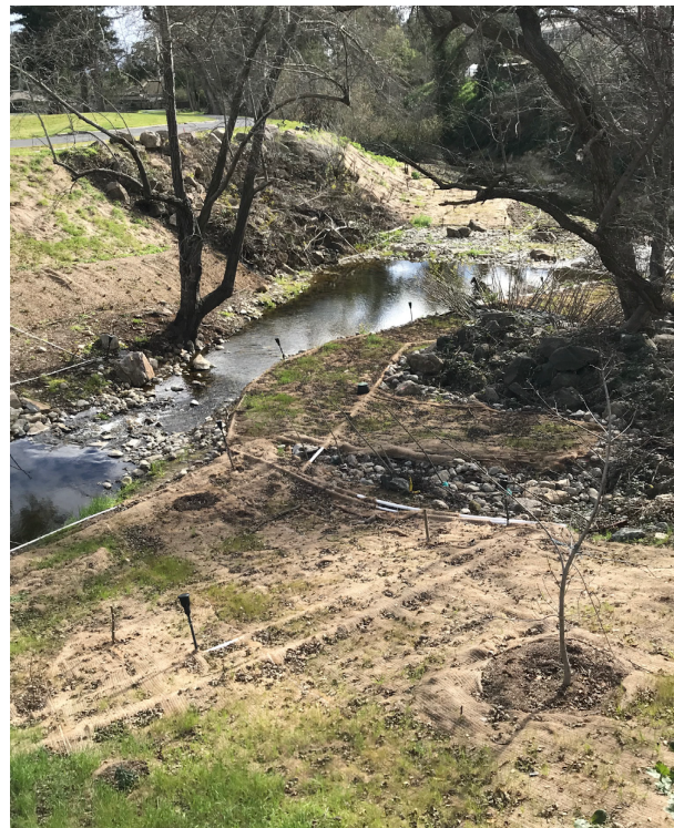
Slope Stabilization and Stream Regrading to Provide Easy Passage for Anadromous Fish
