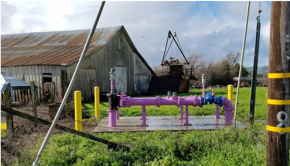
Recycled Water Redistribution System for Agricultural Irrigation Standing Proudly Purple in the Landscape
