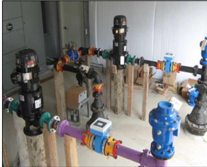
Sunnyvale Upgraded Treatment Plant
