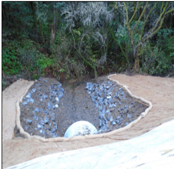
New Culvert Outfall Erosion Stabilization
