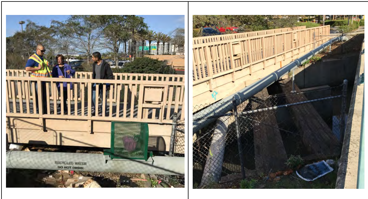
Project Engineer An Bartlett and DWR's Mehdi Mizani discuss construction challenges.
