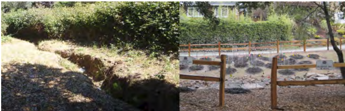
Boyle Park Creek before and after restoration
