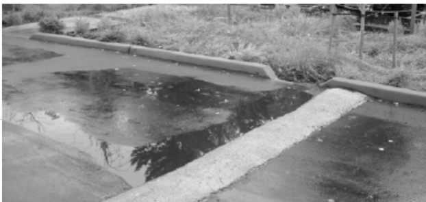
Berm/speed bump was designed to direct water into the bioretention facility
