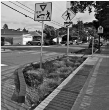
Green infrastructure stormwater treatment facility, City of San Mateo
