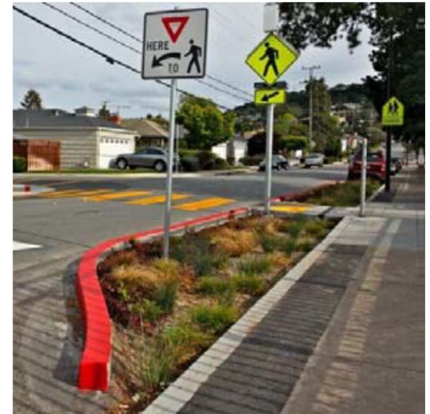
Green infrastructure stormwater treatment facility, City of San Mateo
