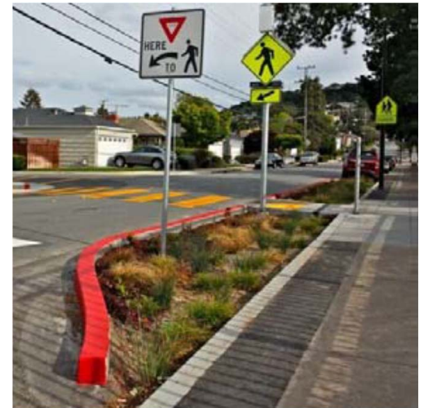
Green infrastructure facility removes pollutants from road runoff
