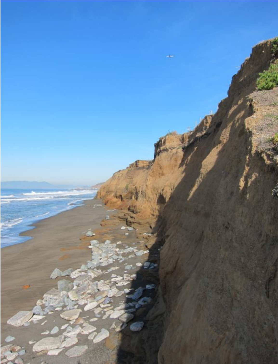
Figure 9: Exposed wave-cut rock platform with scattered riprap at the bluff-beach interface, Pacifica
