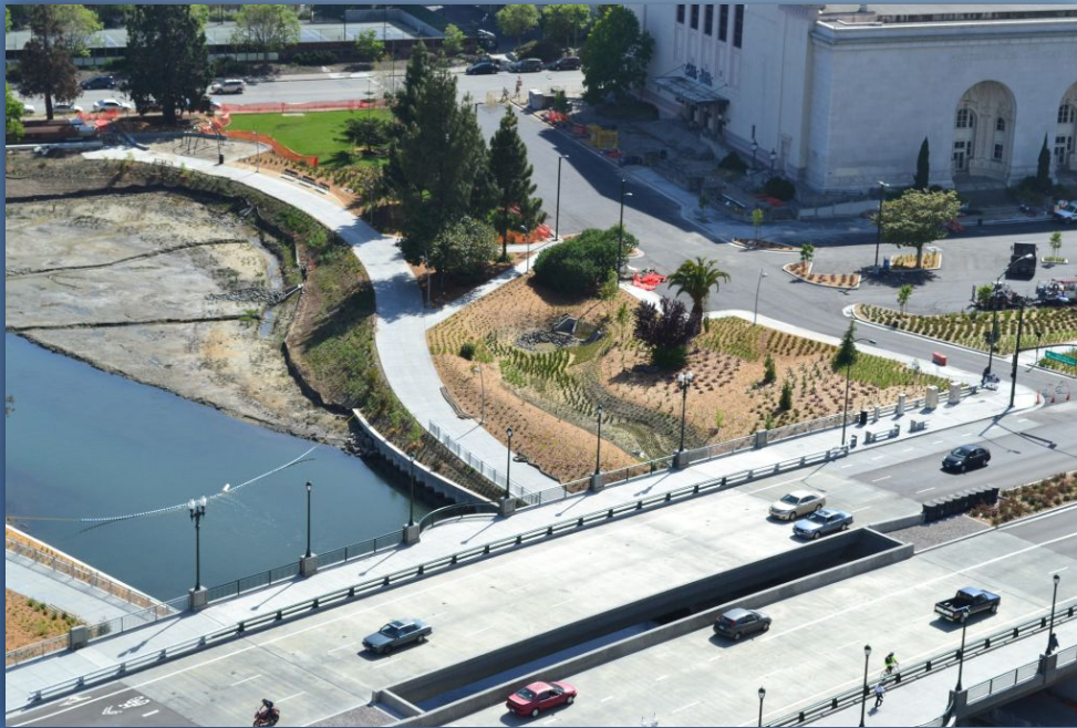
Bioretention at Lake Merritt – May 2013
