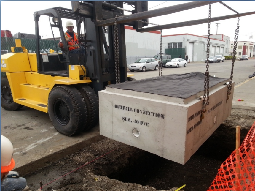
Proprietary Tree Well Installation
