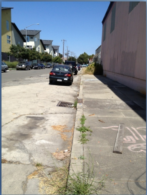
Tree Well Site Pre-Project
