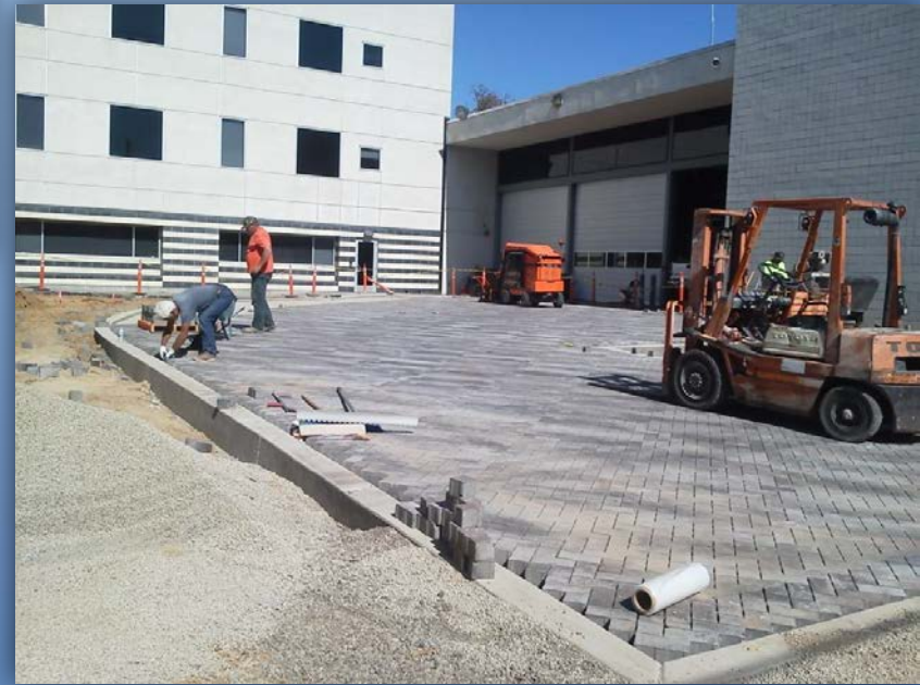
Fire Station 1 Parking Lot Biotreatment Retrofit
