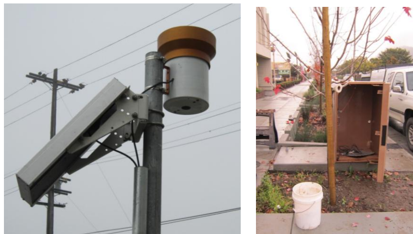
Figure 3.3.2. (A) Rain gage and the solar panel (to charge the battery for the data logger). (B) The lock box (empty, with door open) that housed the battery, data logger, and the ISCO automatic sampler.
