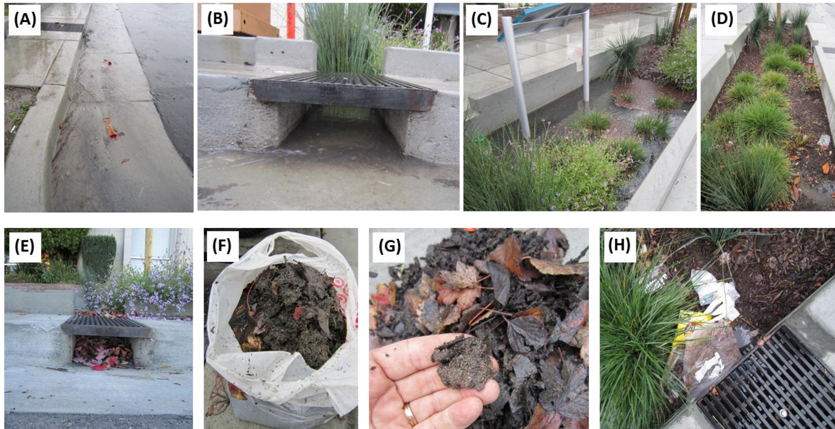
Figure 4.3.2. WY 2011 hydrologic monitoring observations. (A) Flow entering the inlets during the 12/5/10 storm. Local intense bursts of rain can cause high volumes of runoff from the impervious drainage area. (B) Unobstructed flow entering the monitoring cell inlet during the 2/19/11 rain event. (C) Ponded cell with educational sign installed during the 2/19/11 rain event. (D) More southern cell that is not ponded during the 3/13/11 rain event. (E) Accumulation of leaves found in each inlet, necessitating early season maintenance as a critical component to performance (11/2010). (F) Material (sand and organic debris) removed from the monitored inlet after the 12/5/10 storm. All of the inlets accumulated material; however the monitored inlet had the largest deposit because it is the furthest “upstream”. (G) Sand-sized deposits removed from the inlets. (H) Example of food wrapper trash commonly found in the garden.
