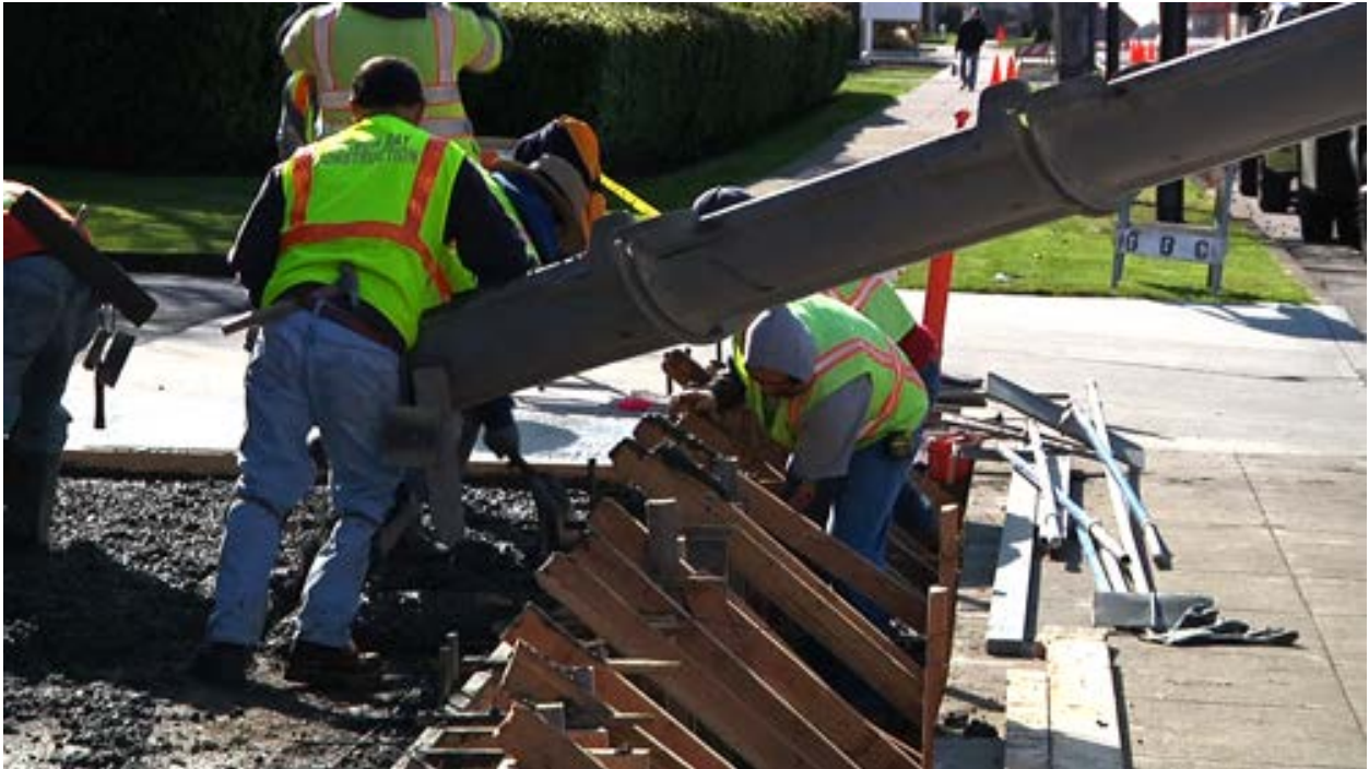
10 Pouring concrete for new sidewalk, Madison site
