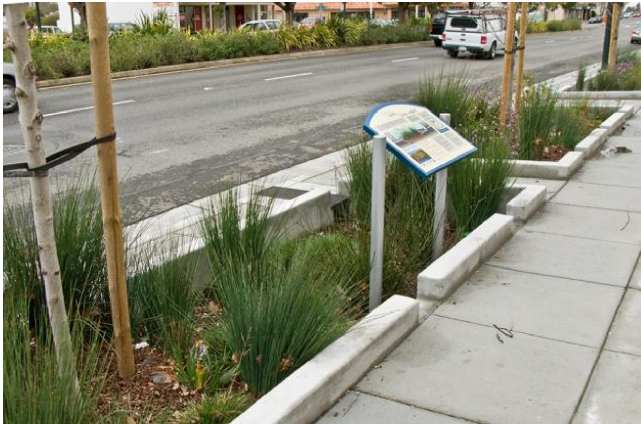
26 Eureka site, looking north, 1 year post-construction (March 2011)
