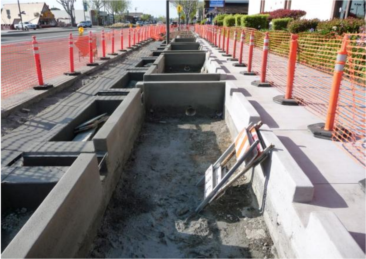
11 Formed rain garden cells, Madison site
