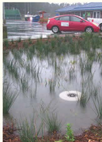
This rain garden in Daly City treats polluted water from an adjacent parking lot. Photo above and below by SFEI.
