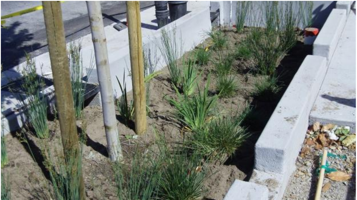
14 Close up of newly installed plantings, site unknown
