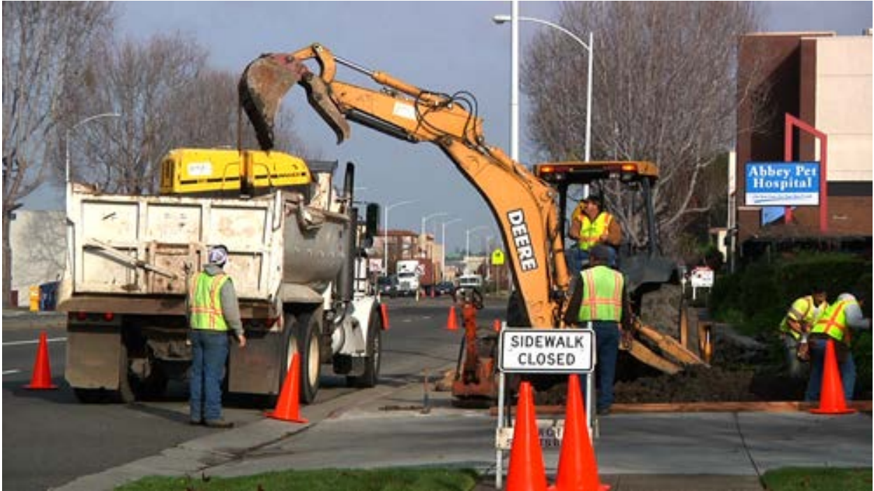
9 Loading Spoils for disposal, Madison site
