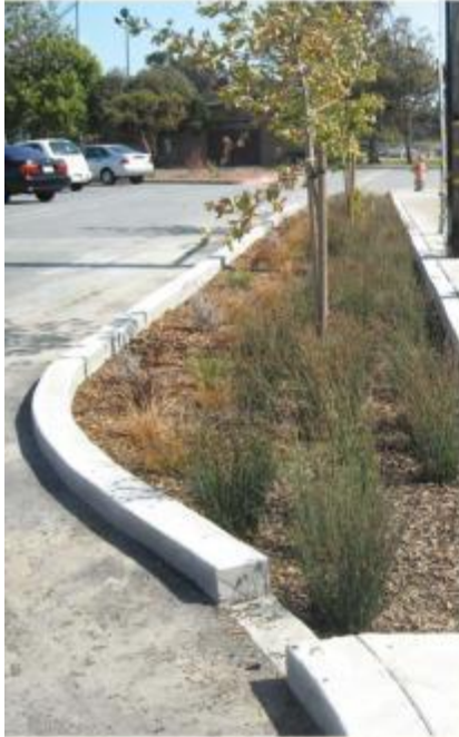
Stormwater from the street flows into this curb extension in San Bruno.
