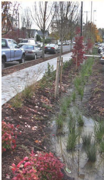
This bioswale filters runoff from the adjacent parking lot. Photo courtesy Kevin Robert Perry.
