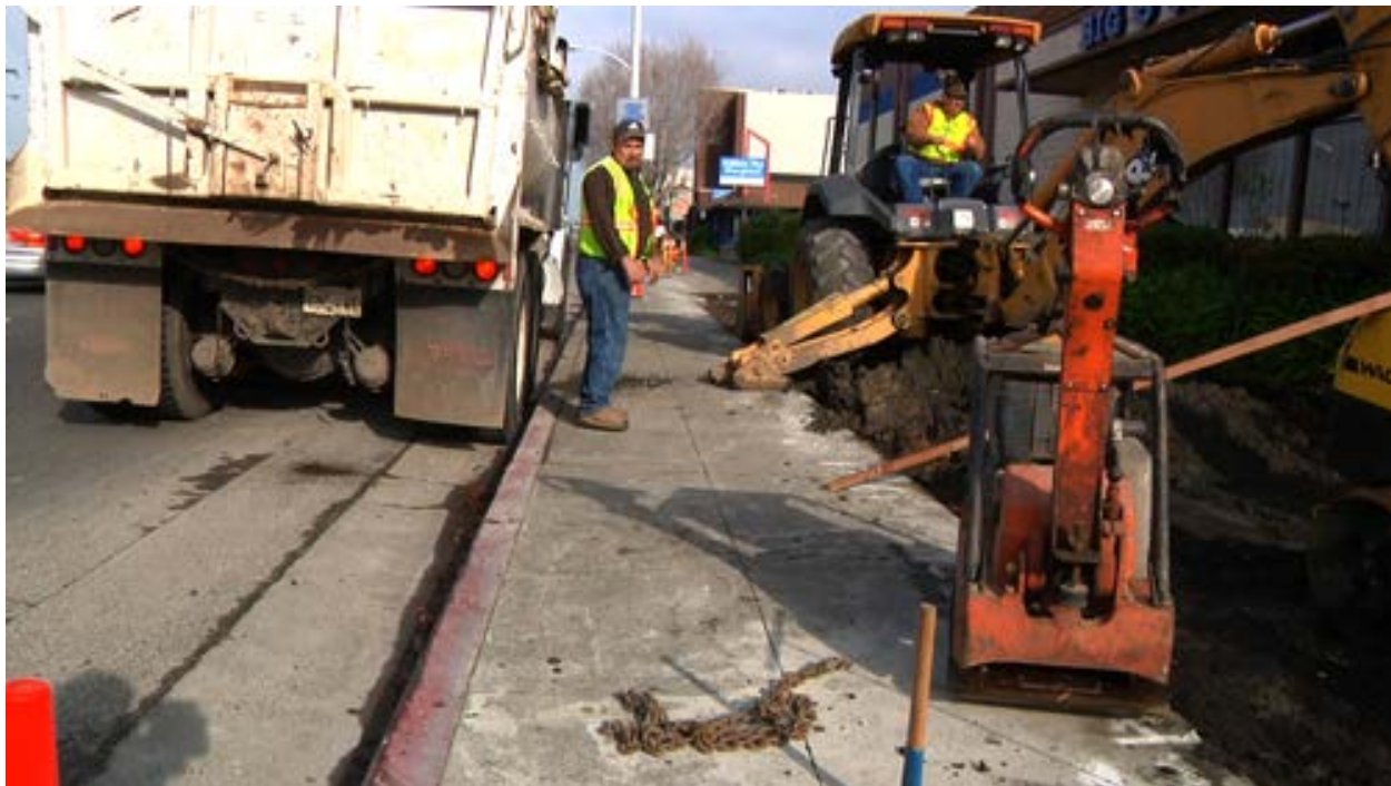
8 Excavation, Madison Site
