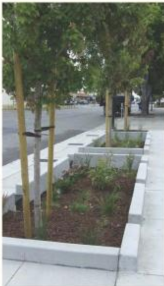
The El Cerrito planters were built below grade so that polluted water running off of the street and sidewalk will flow into them and be filtered before going into the storm drain system and the Bay. Photo by Lisa Owens Viani.
