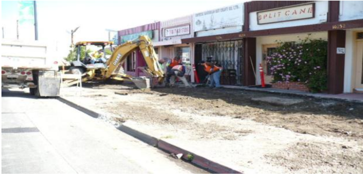
7 Sidewalk removal, Eureka site
