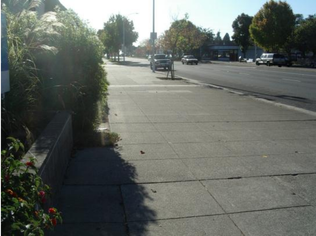
22 Madison site, pre-construction, looking south
