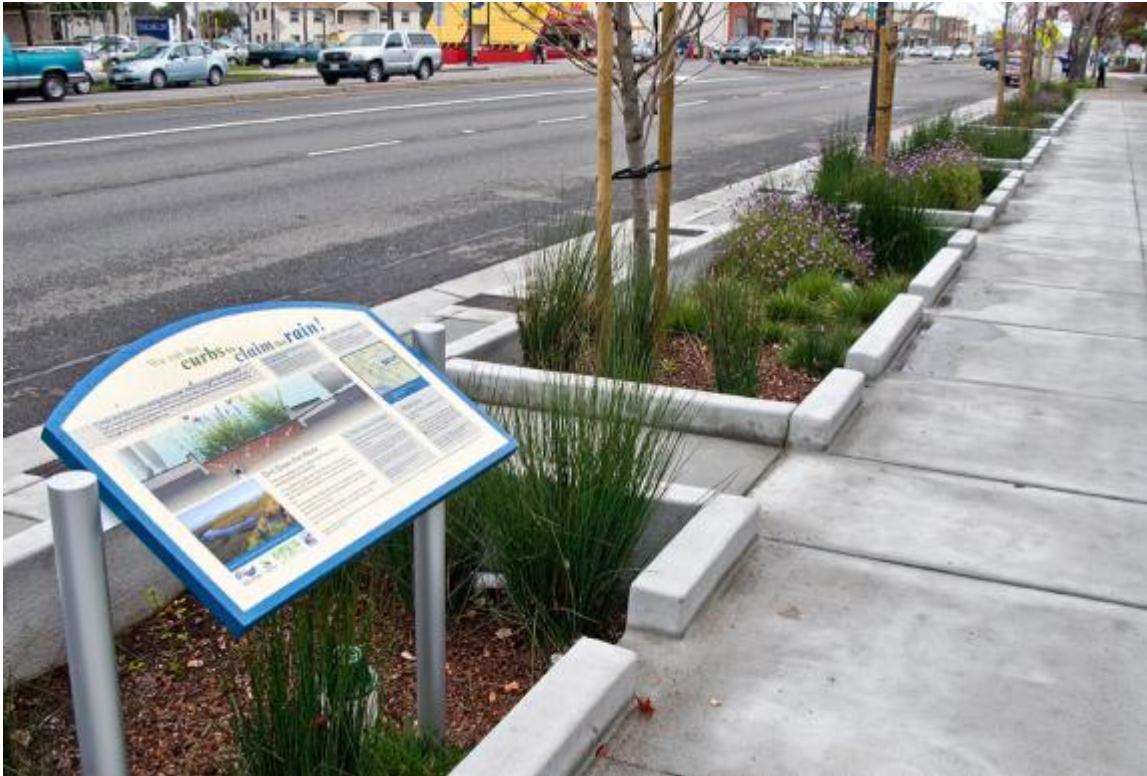
24 Madison Site, looking north, 1 year post construction (March 2011)
