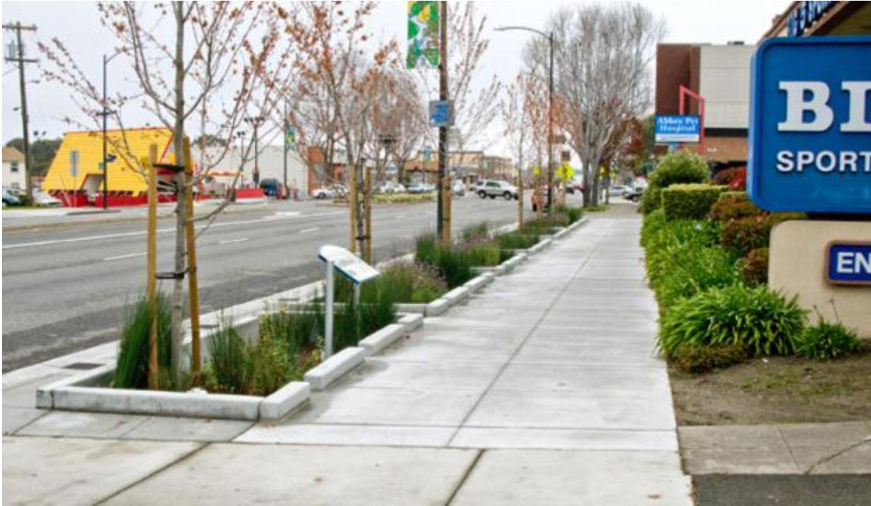
23 Madison Site, looking north, 1 year post-construction (March 2011)
