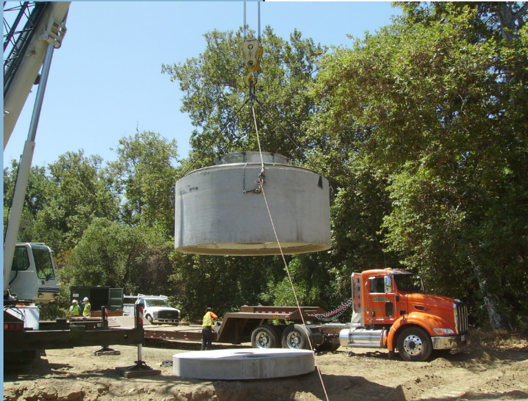
Installing a large trash capture device, San José
