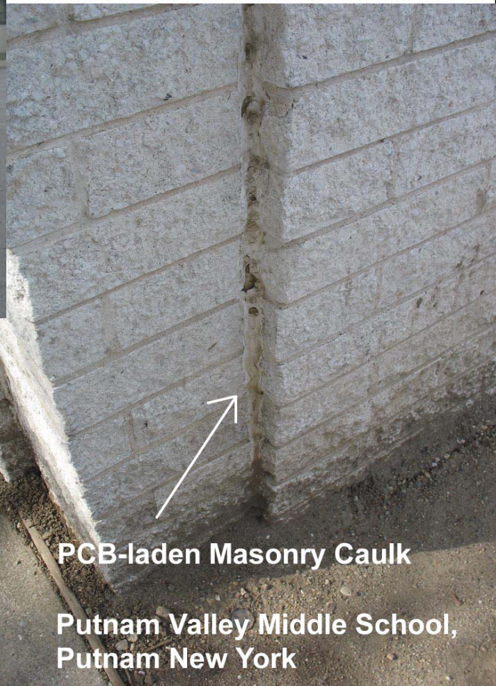
PCB-laden masonry caulking on exterior wall. Putnam Valley Middle School in Putnam NY
