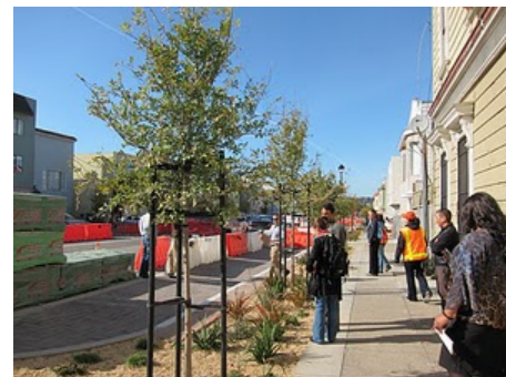
Newcomb Avenue stormwater infiltration area
