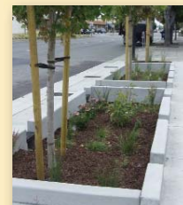
Stormwater planters are being installed along the East Bay's San Pablo Avenue corridor.
