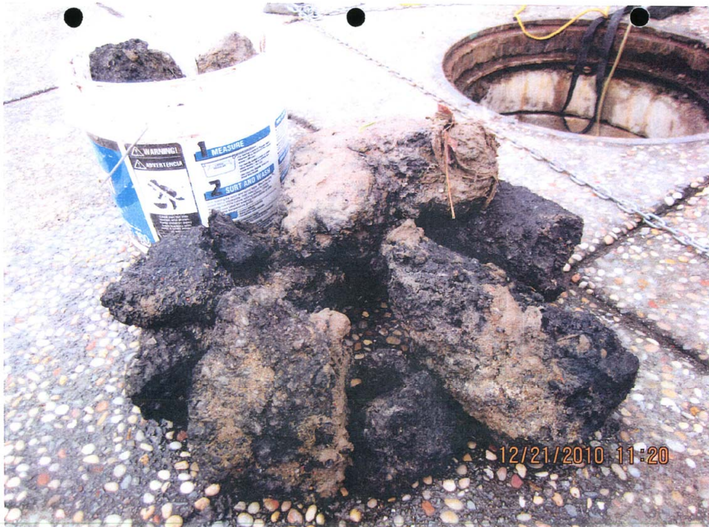
Photo 1: District photo of construction debris removed from the 27-inch Kent Middle School pipeline at manhole #2513 on December 21, 2010 at 11:20 am.
