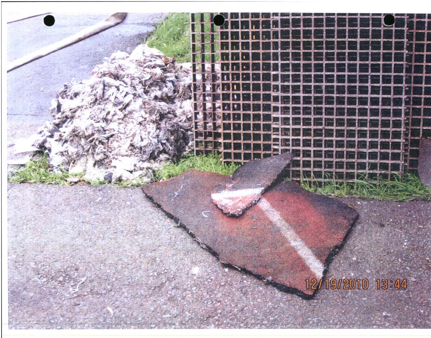
Photo 3: Nute Engineering, Inc. photo of December 22, 2010, SSO, from manhole #2647 at the intersection of Behrens Drive and Sherwood Ct.
