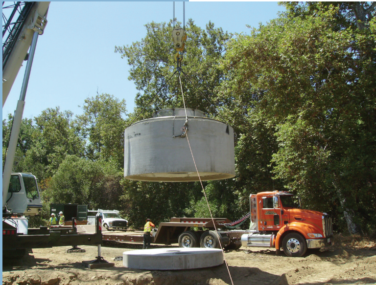
Installing a large trash capture device, San José
