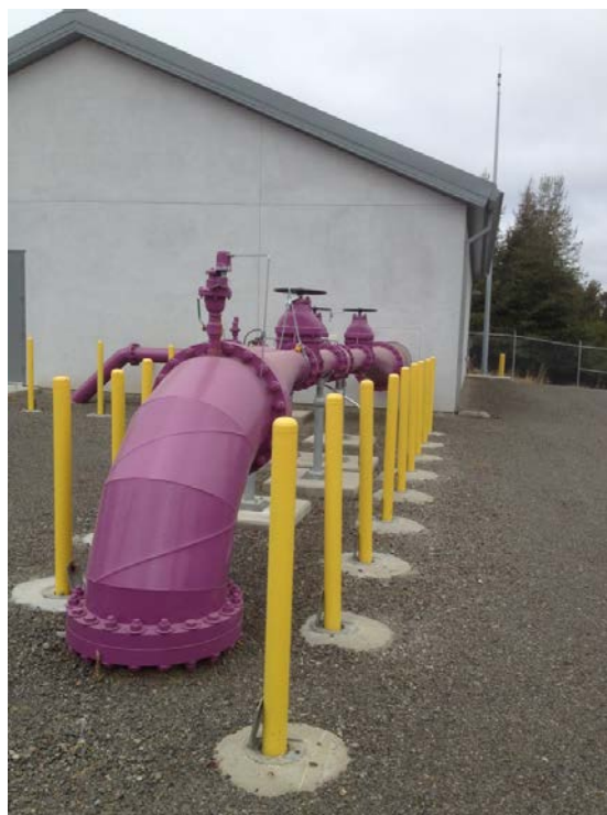
MST recycled water distribution line at new pump house.
