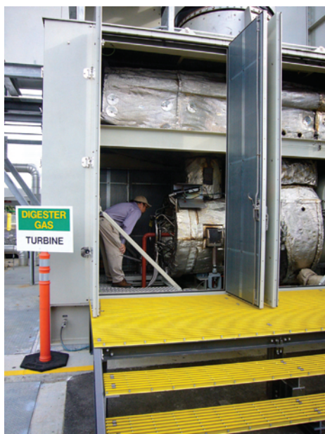
EBMUD’s innovative new turbine, which produces enough electricity to power 5,000 homes. Photo by Ariel Okamoto.
