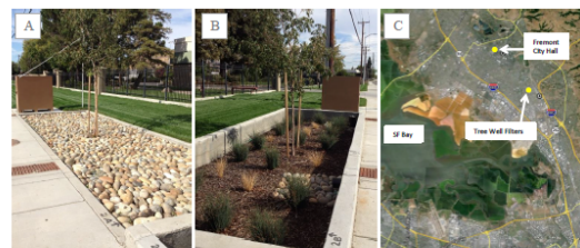
Figure 1. A) Subsurface-loaded tree well filter, B) surface-loaded tree well filter, and C) regional aerial of southeast South San Francisco Bay showing location of tree well filters in the urban Fremont area.
