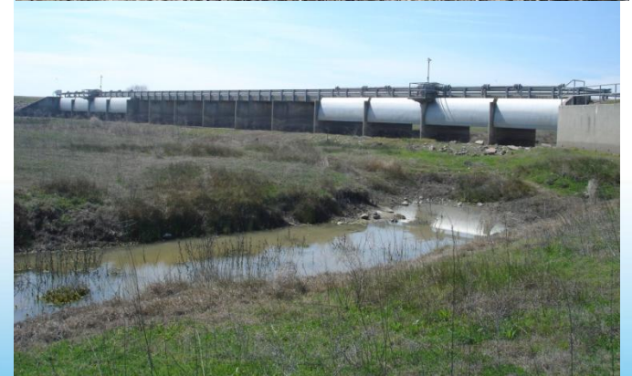
Mariposa Bypass gates, San Joaquin River, CA
